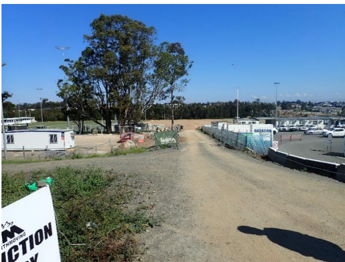
Figure 17. Northern end of the study area showing work-site compounds, carpark and eucalypt trees, looking west
