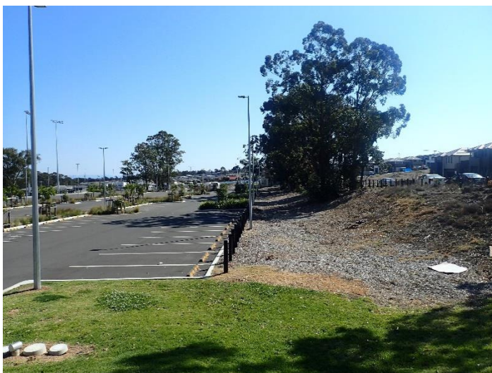
Figure 14. The carpark and eastern embankment, looking north-west
