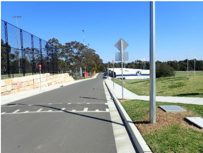
Figure 16. The southern boundary of the study area showing services along the pathway and building in the background, looking west
