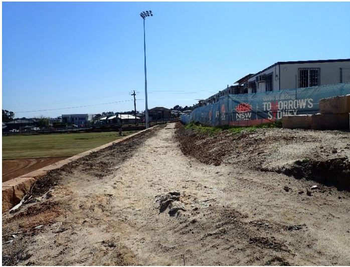
Figure 18. Western boundary of study area showing sandstone retaining wall, looking north
