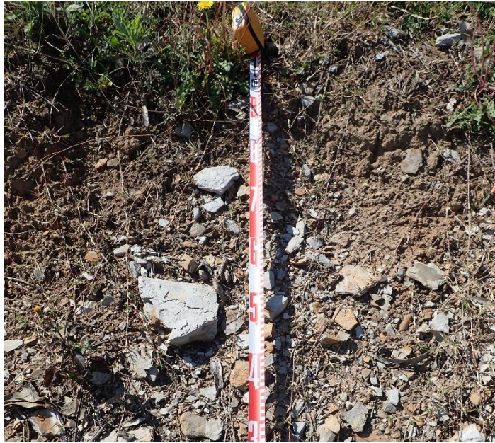
Figure 15. Exposed ground on the eastern embankment showing redeposited clay and shale and pieces of road gravel, looking east
