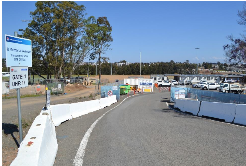
Figure 15. The road works compound in the north of the study area, looking west
