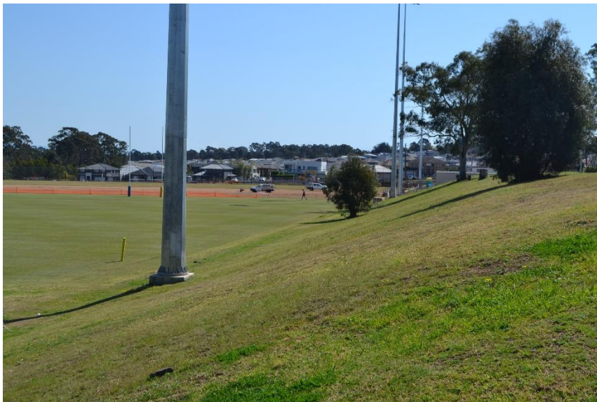
Figure 10. The embankment between the playing fields and the carpark, looking north
