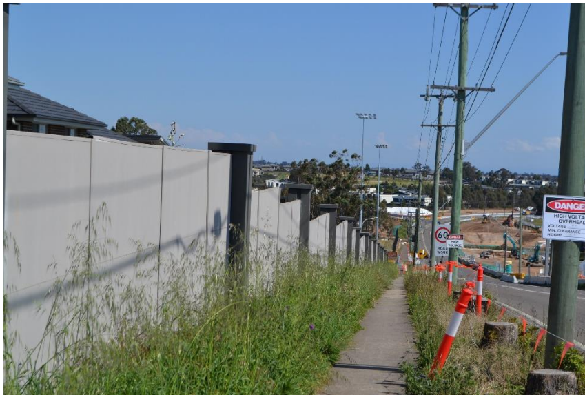
Figure 19. Looking west along Memorial Avenue, from Windsor Road towards the study area
