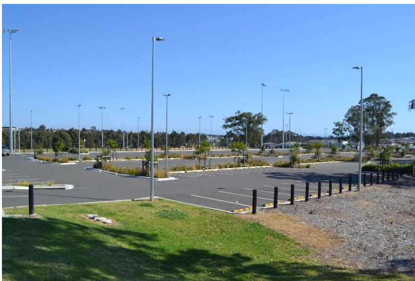
Figure 11. The carpark, looking north-west
