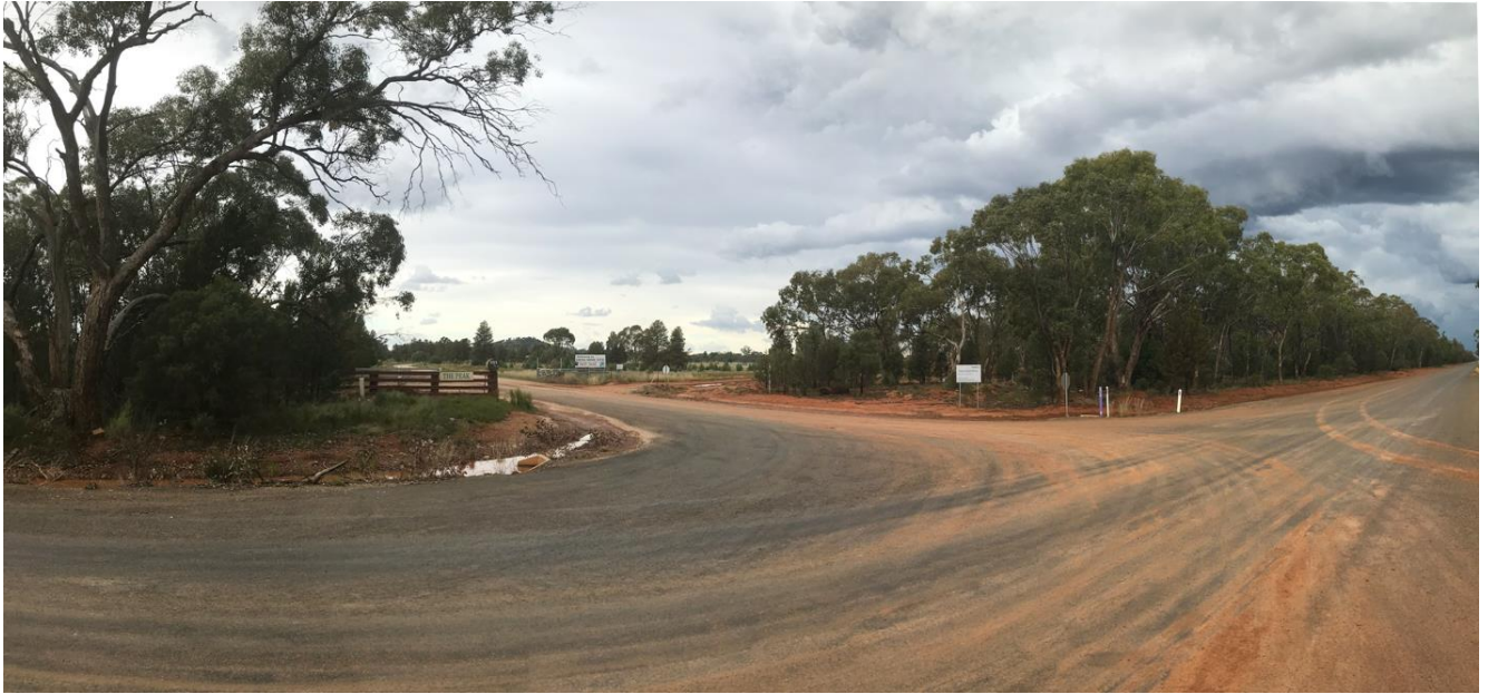
Photo 1 VP1 - Existing Hera Mine Entrance
