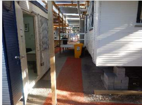
Figure 17: Temporary construction workers' building on brick pillars over levelled ground. View South
