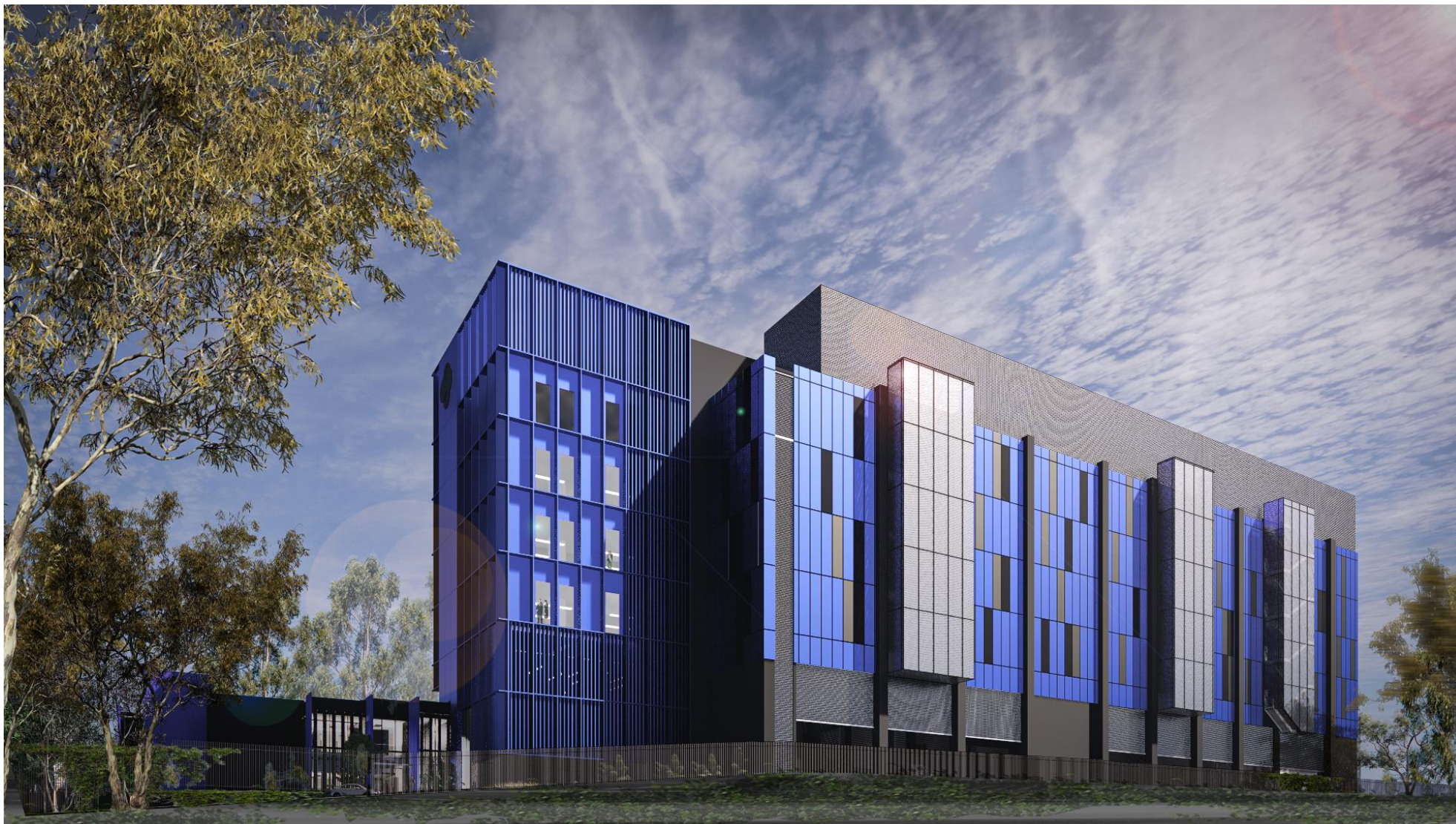
Figure 12 Indicative view of building from west (Source: HDR, 2021)
