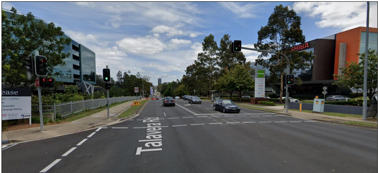
Figure 7 Street view looking north-west from Talavera Road towards subject site (Source: Google, 2020)
