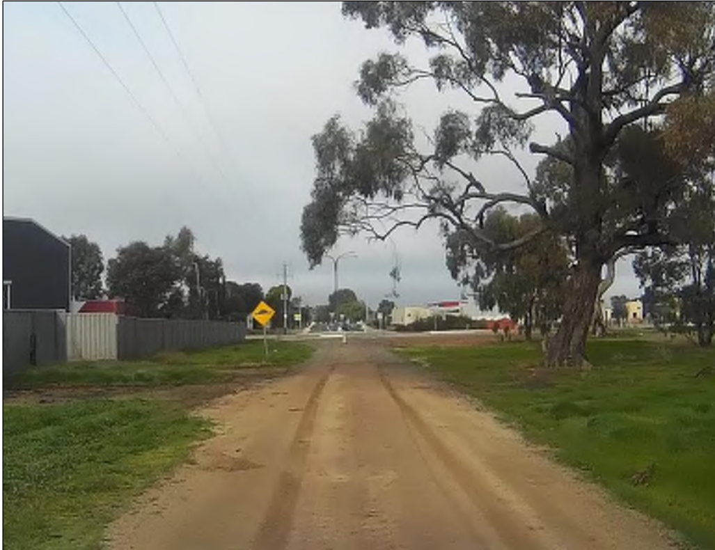
Photo 7: Kirchhofer Street looking south
