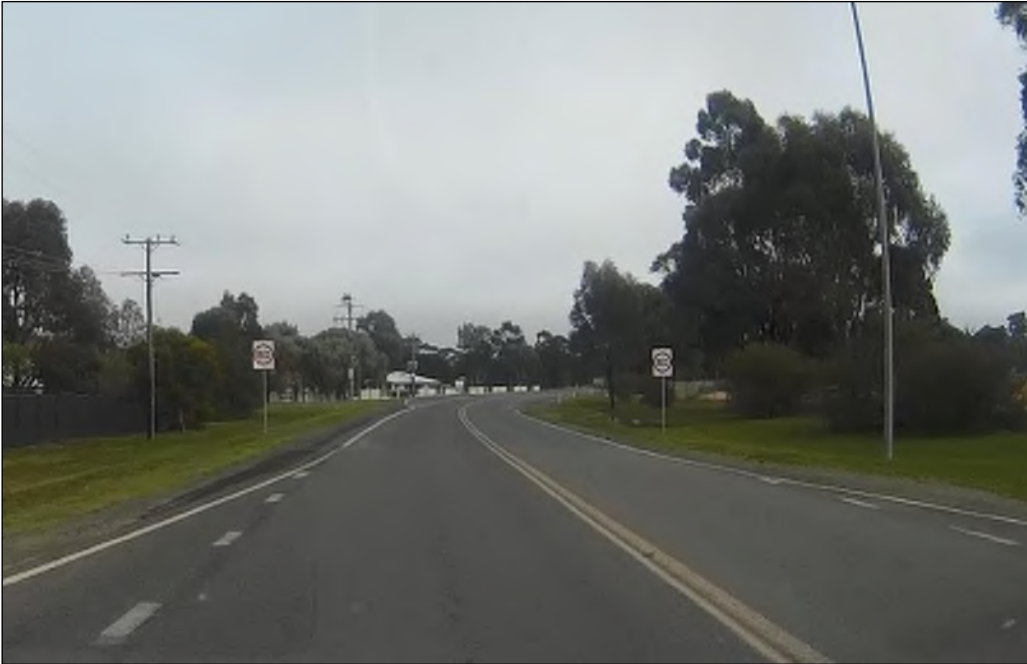
Photo 3: Perricoota Road looking west
