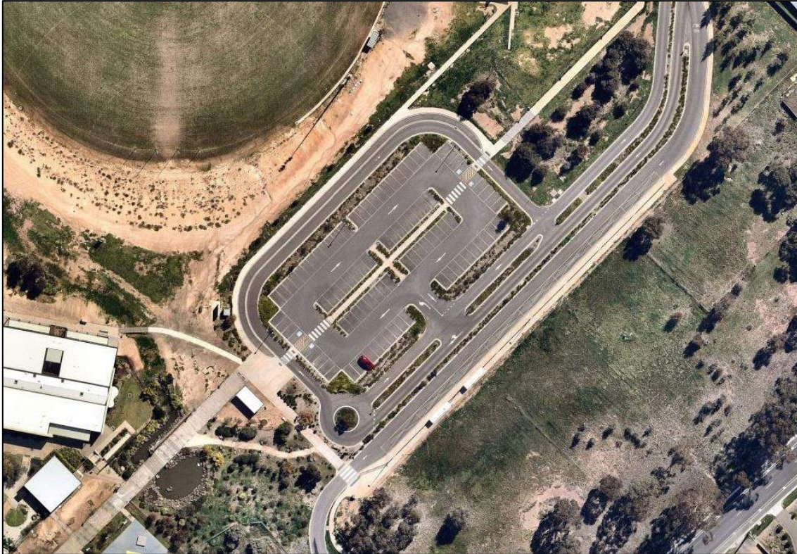
Figure 9: Marist College drop-off/pick-up car park
