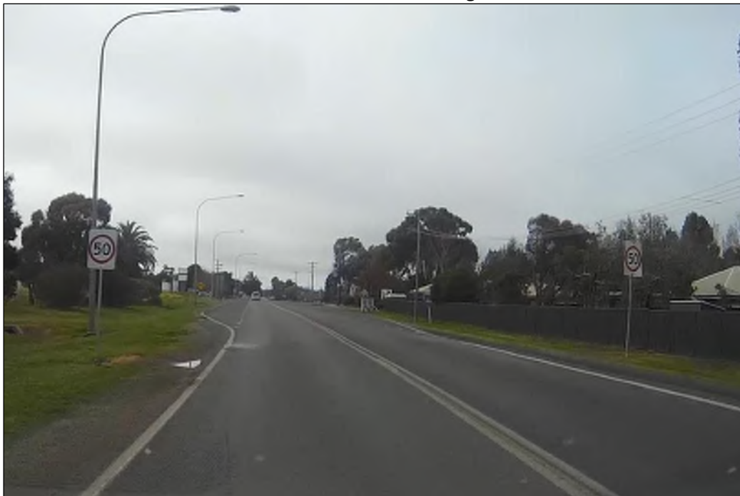
Photo 4: Perricoota Road looking east
