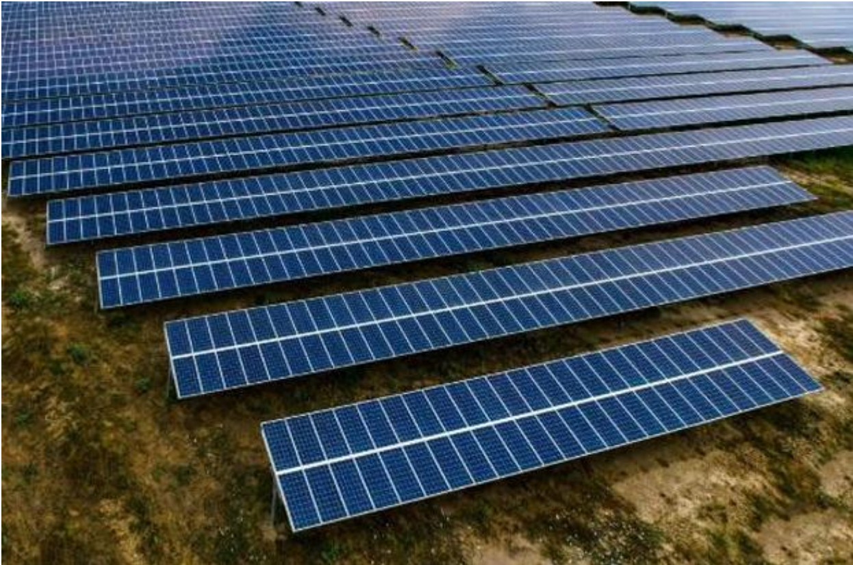
Photo 1.1 Typical 2P solar panel mounting
