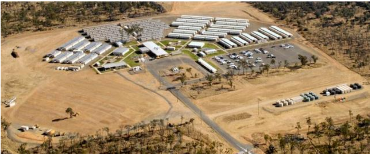
Photo 1.3 Typical Temporary Workers Accommodation Facility
