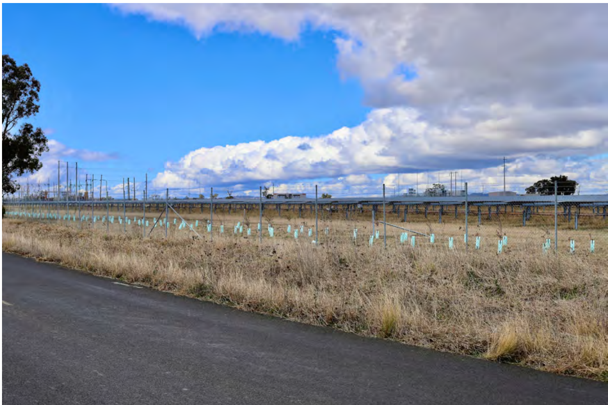
Figure 7-3: Photograph of Beryl Solar Farm, taken from Beryl Road (immediately adjacent the solar farm)
