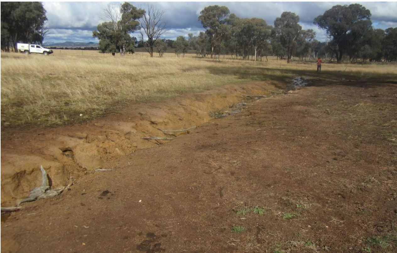
Photo 4.3 Eroded drainage line within the Amended Project Area Located near the middle of the west boundary to the Amended Project Area.
