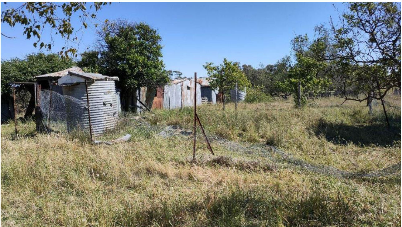
Photo 4.7 Ancillary structures and shed associated with the c.1900s cottage
