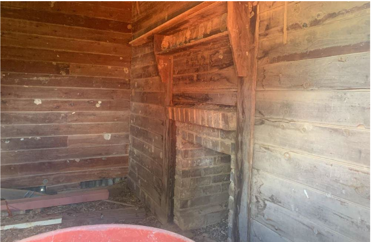
Photo 4.9 Fireplace and timber boarded walls within the c1870s hut
