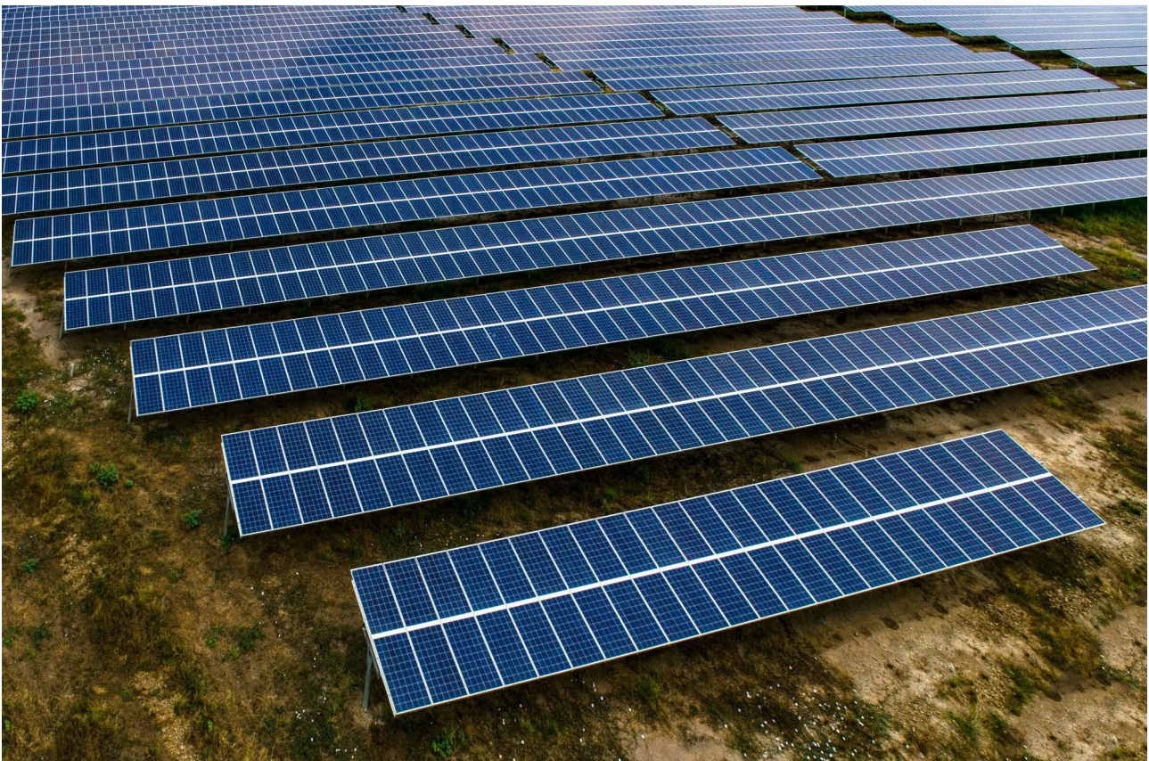
Plate 2.1 Example of 2P solar panel mounting
