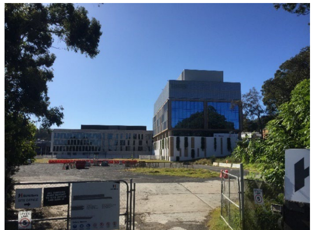
Picture 4 – Looking north from existing site entrance
