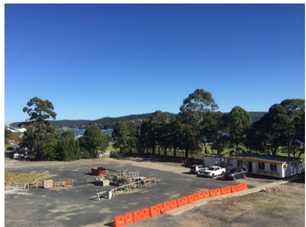
Picture 6 – Looking south at site from Mann Street
