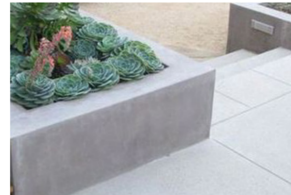
CONCRETE RETAINING WALLS (W1)
