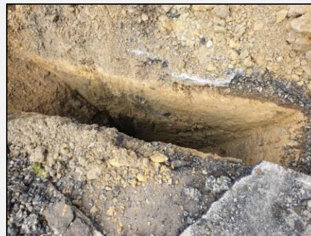
Photo 4: Overlying fill material observed at TP2.
