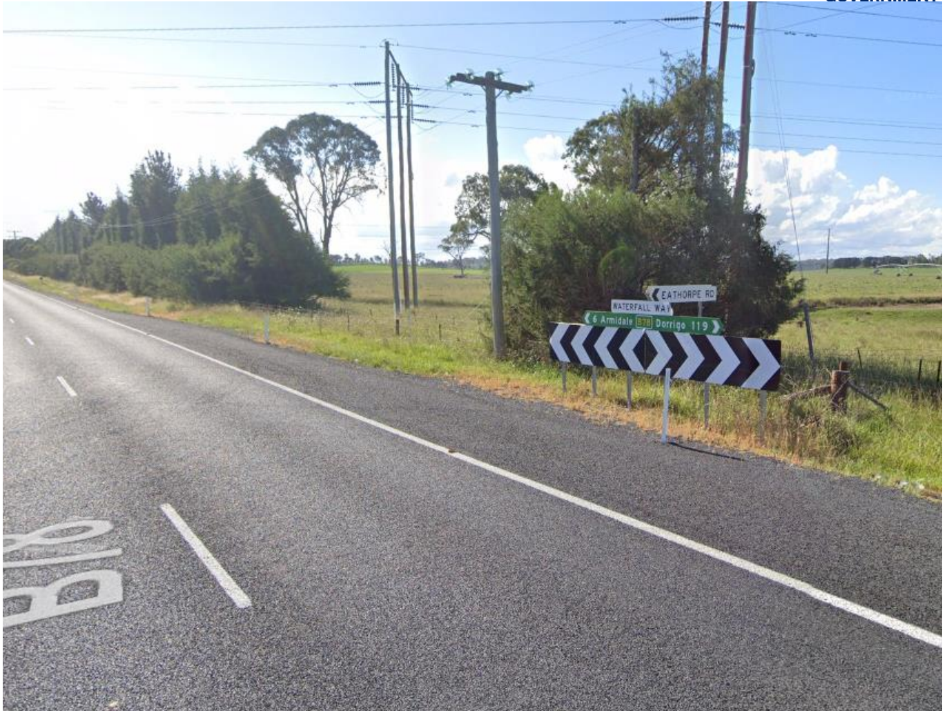
Figure 7: Example of power pole hazard on northern side of Waterfall Way at its intersection with Eathorpe Road.
