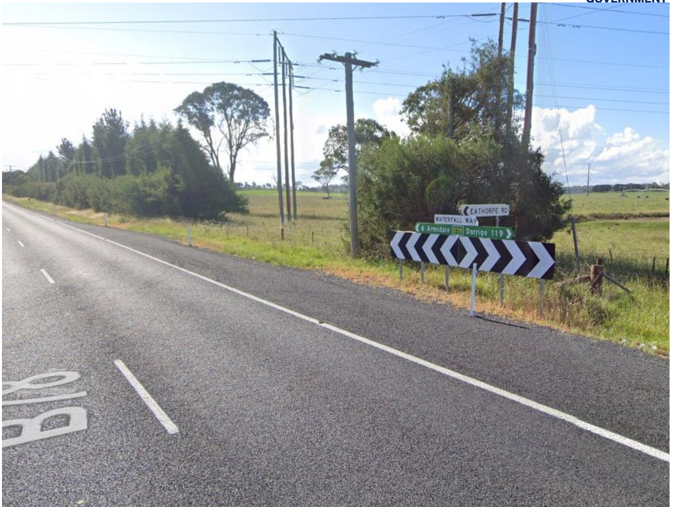
Figure 7: Example of power pole hazard on northern side of Waterfall Way at its intersection with Eathorpe Road.
