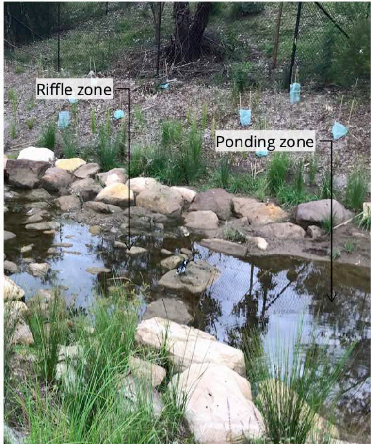
01 CHANNEL DETAIL PLAN - SCALE: 1:400@A1 Channel Design Precedent Image
