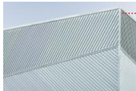
Colorbond Metal Sheetting 'Dover White' – Translucent sheeting effect for warehouse 2 (temperature controlled space)
