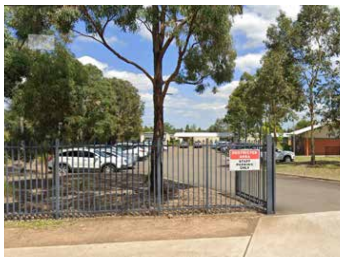
Figure 14. View of the existing staff entry and carpark accessed from The Ponds Boulevard
