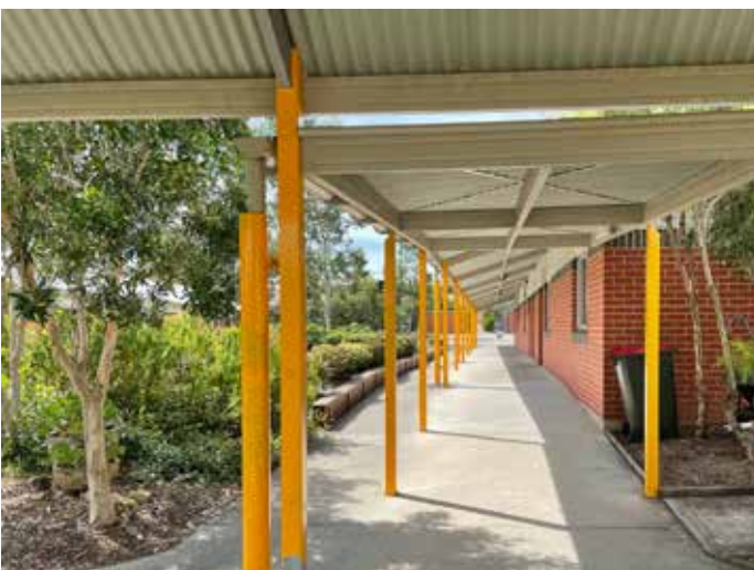
Figure 7. View of covered walkway
