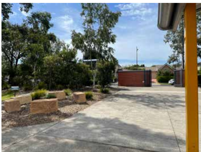
Figure 13. View of the pedestrian entry to the school looking towards The Ponds Boulevard
