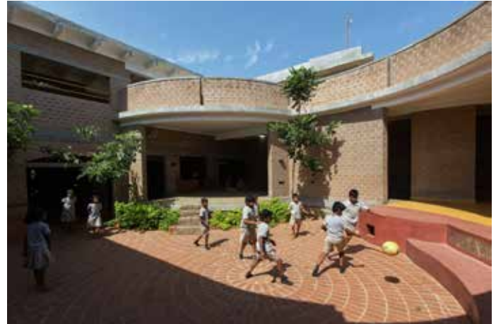
Figure 25. Yellow Train School - outdoor space and amphitheatre
