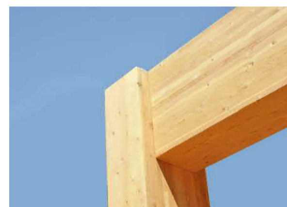
GLT Frame Glue Laminated Timber (GLT)for internal framing
