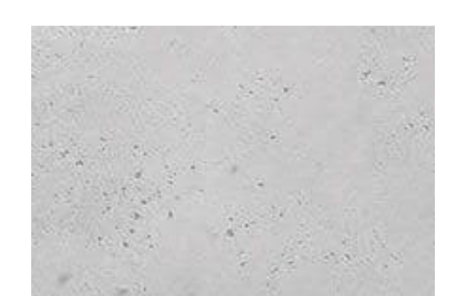
CON-101 Concrete framing Keim finish for longevity and quality
