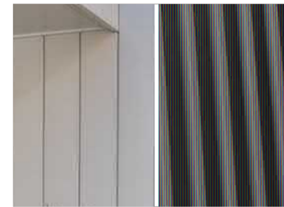
CLG-301 CLG-302 Dominion and SnapSeam for Soffit Linings (Standing Seam) Colour TBC
