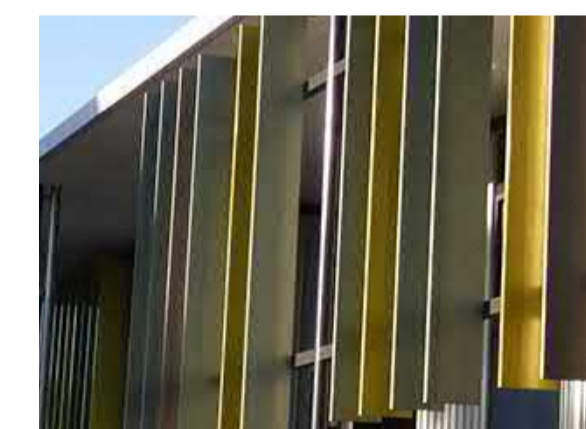
SCN-102 Arcadia Louvres Aluminium Extruded box section aluminium Colours to be confirmed
