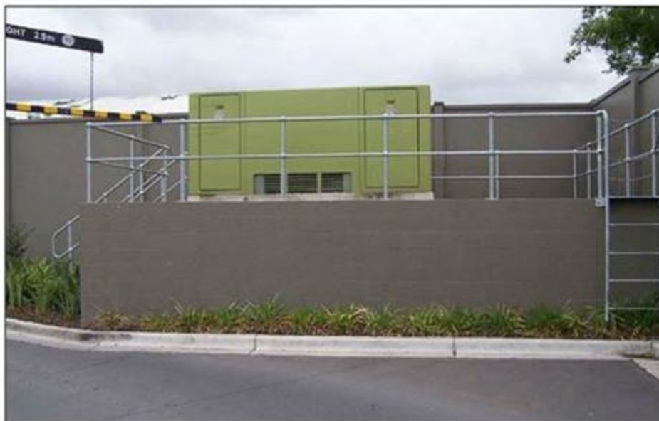
Figure 51 - Example substation raised above 1:100 flood level
