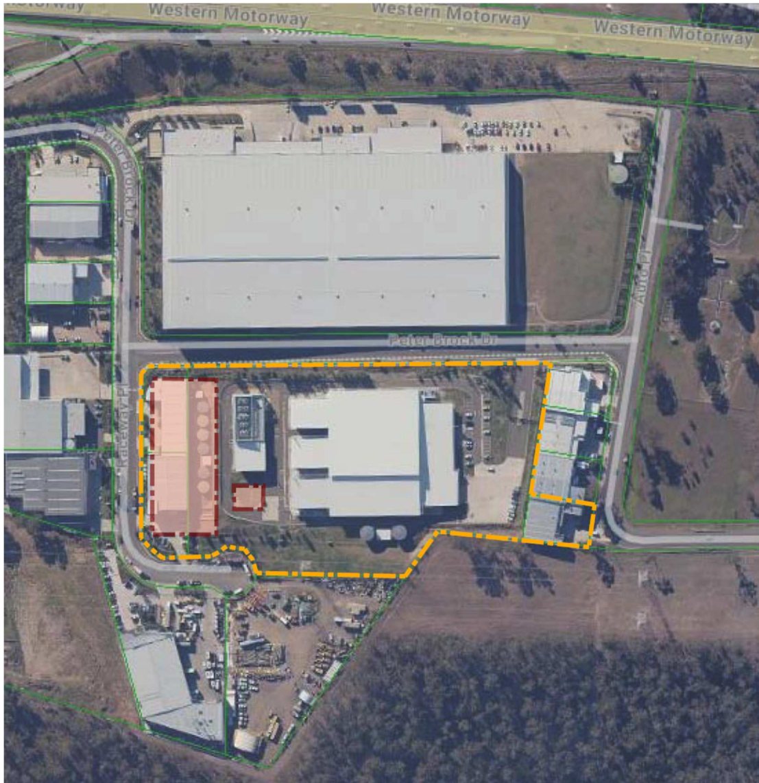
Figure 18 – Aerial Photograph of the Data Centre Site and adjoining land.
