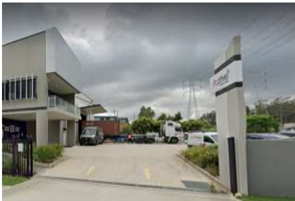
Figure 16: Buildings on the corner of Raceway Place proposed to be demolished
