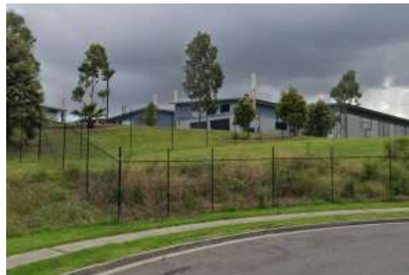
Figure 17: Data centre and terraced landscaping Raceway Place
