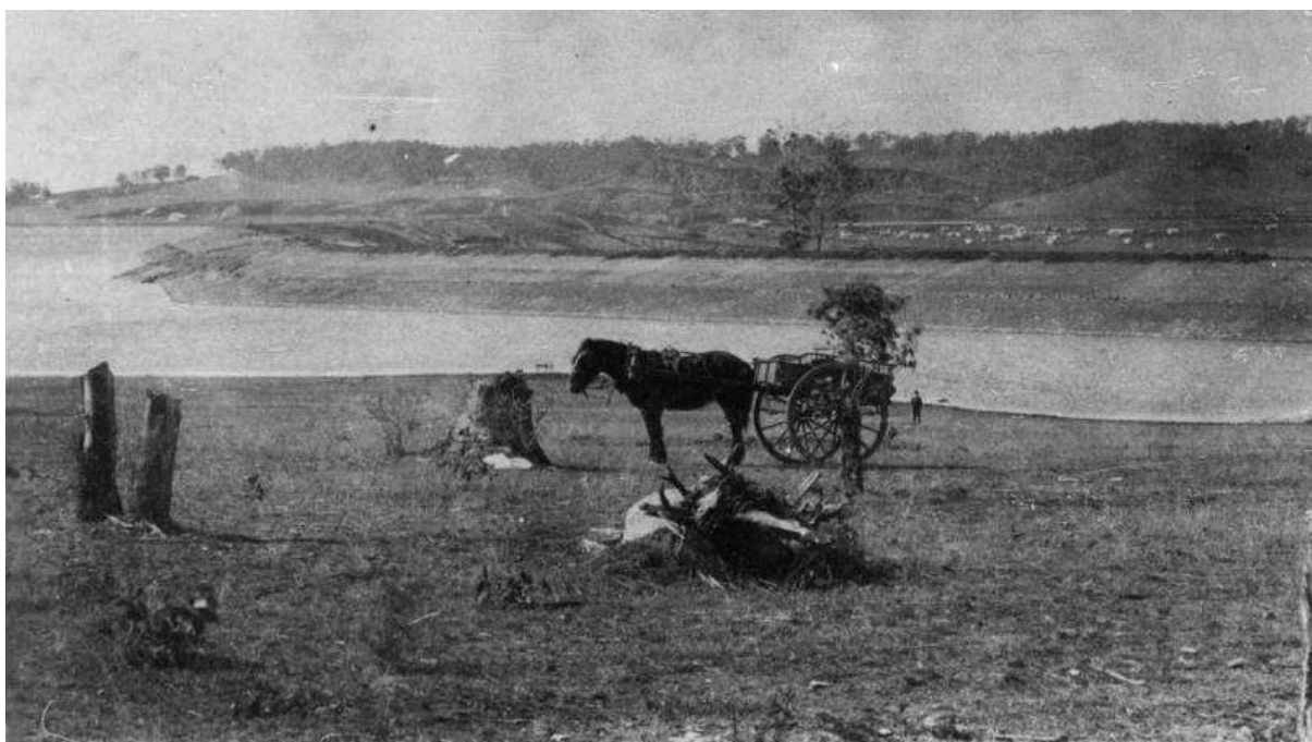
Figure 4: Prospect Reservoir during construction, c1880s (Source: Blacktown City Libraries)
