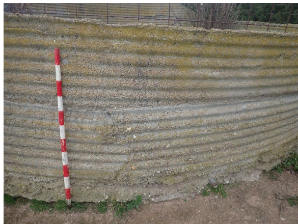
Figure 6-51 Detail of corrugated surface of cement water tank
