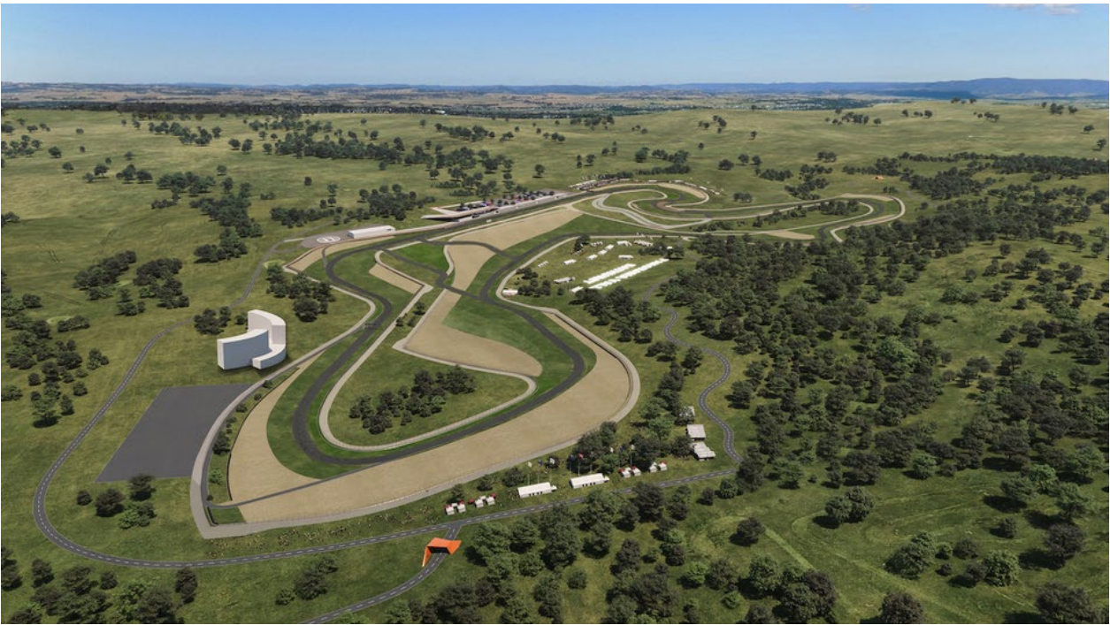
Figure 7-3 Large local developments include the Bathurst Second Circuit, 18km from the Project.
