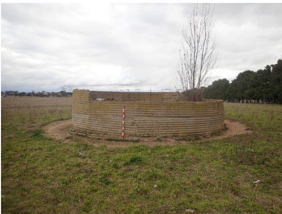
Figure 6-50 Cement water tank in paddock behind Woodside Inn.
