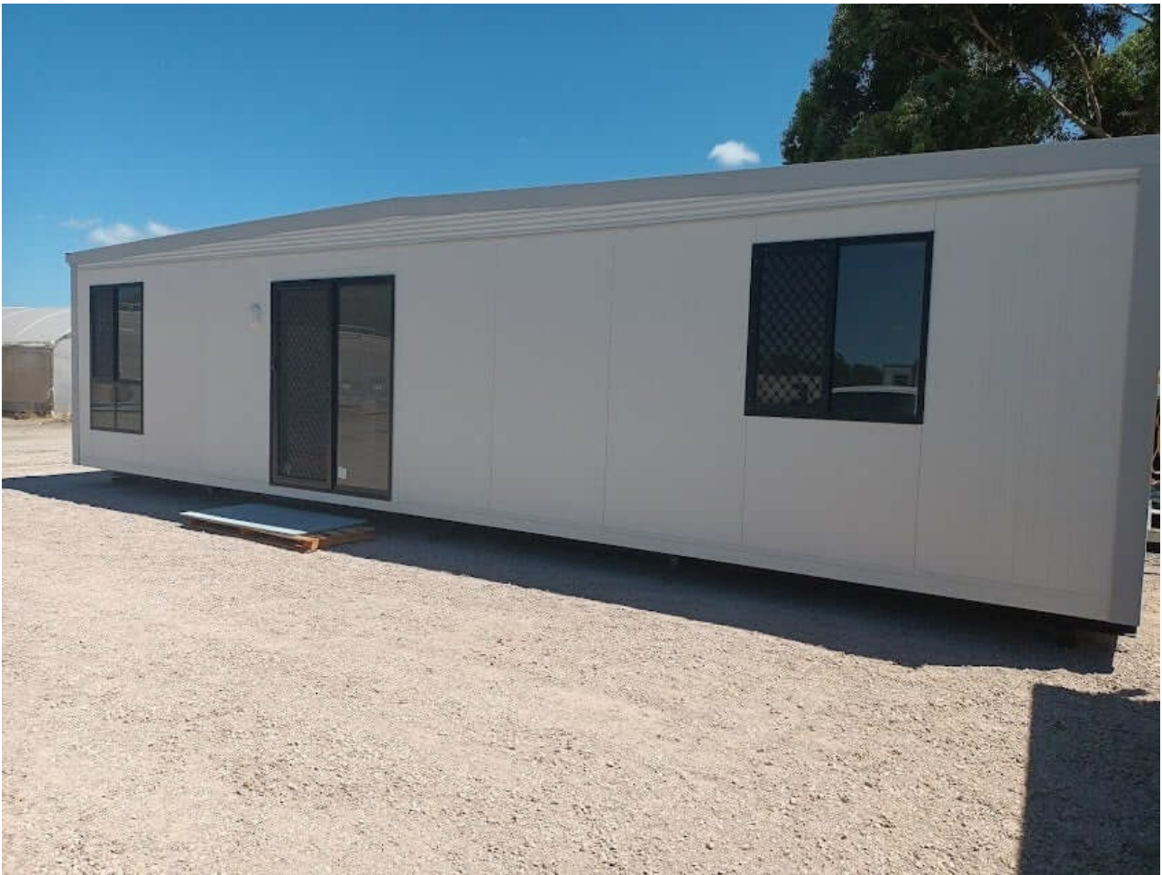
Figure 3-10 Typical construction facilities
