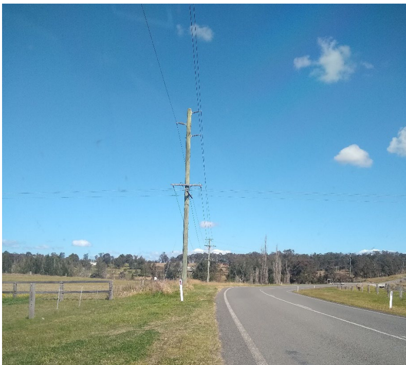
Figure 2-2 Example of an 'underslung' line, applicable to Sections A-B and G-H
