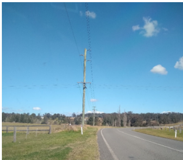
Example of an "underslung line".
