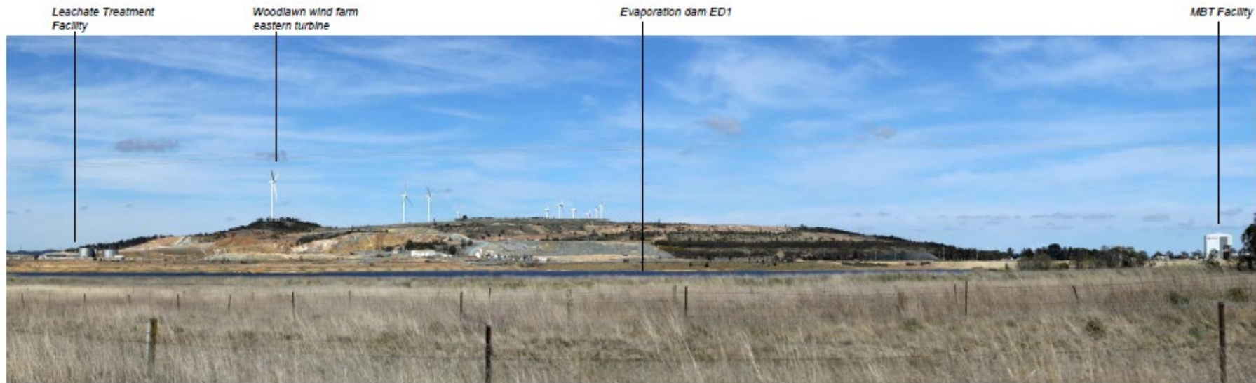
Photograph 8.5 P5 Collector Road. View south-west to south-east toward the Eco Precinct.
