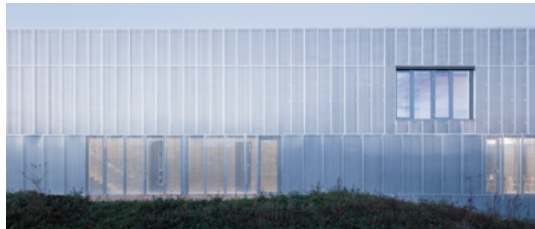
TRANSLUCENT NON COMBUSTIBLE SHEETING
