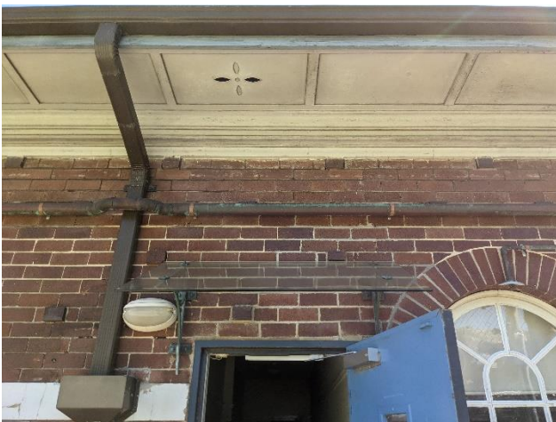
Figure 14 – New door opening at Level 2 south façade and soffit vent detail.
