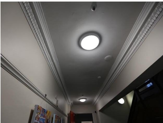
Figure 32 – Cornice in corridor with dentil details.
