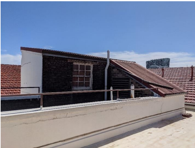
Figure 18 – Staircase overrun
