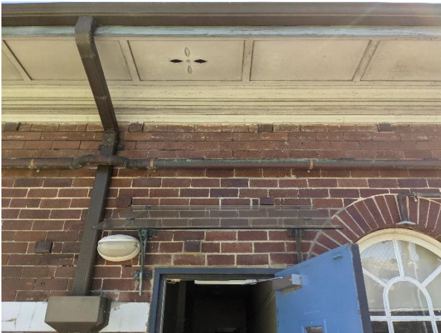
Figure 20 – New door opening at Level 2 south façade and soffit vent detail.
