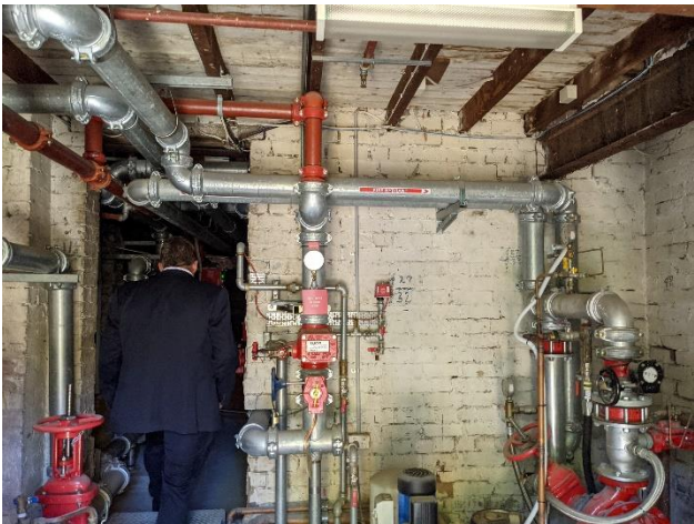
Figure 64 – The sprinkler room
