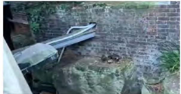
Figure 11 – Natural sandstone bedrock showing extent of excavation with brick wall above and services/subsistence work. Aspect: North east.
