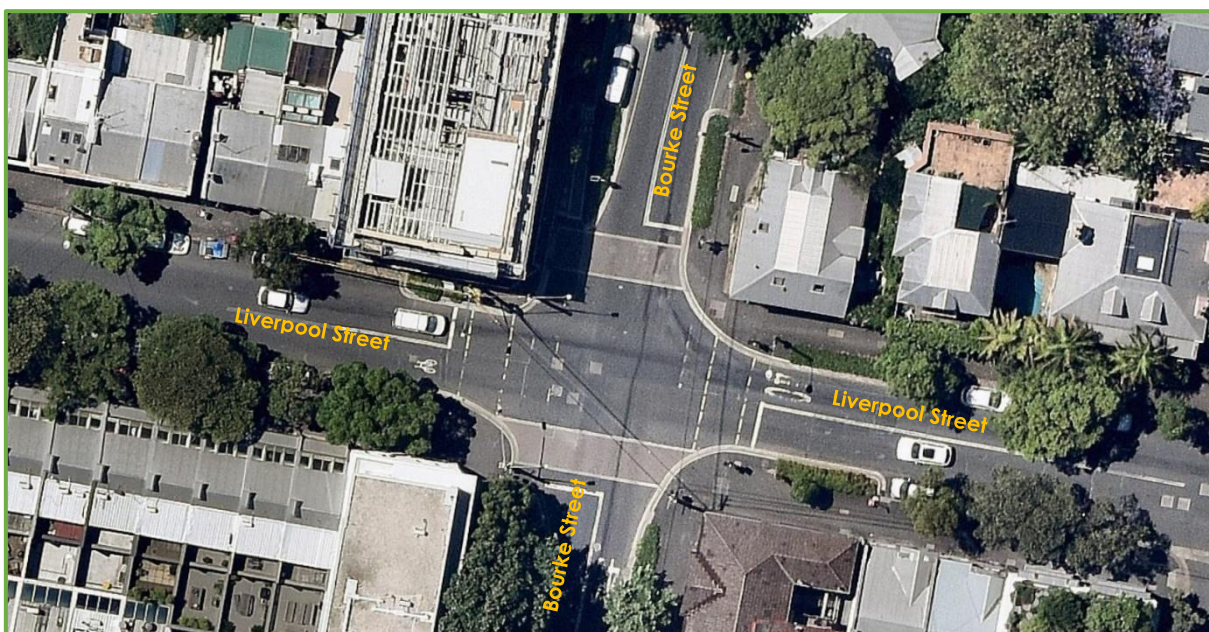
Figure 4: Intersection of Liverpool Street and Bourke Street
