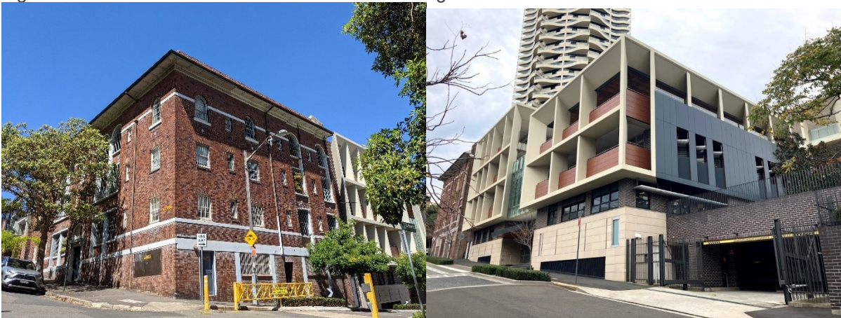
Figure 3 Wilkinson House and Joan Freeman building as viewed from St Peters Street
