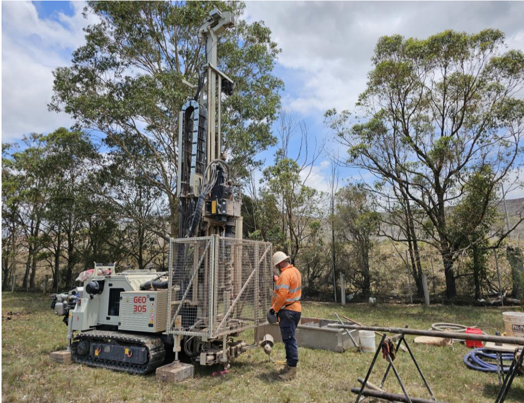
Photo 9 - Typical Drill Rig Set Up
