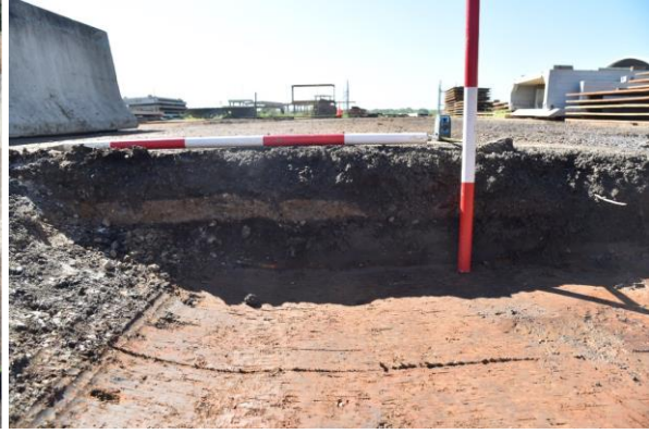
Figure 49: Southeast profile view of TT 5, showing the deposit of grey sand and aggregate (049) between the two asphalt layers at the north end of the trench
