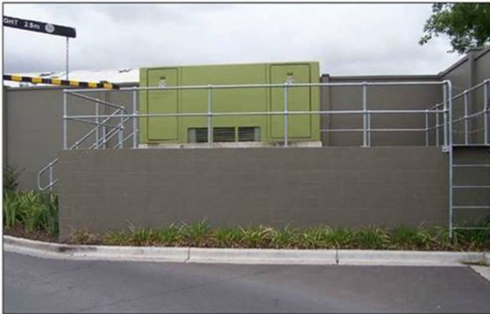
Figure 51 - Example substation raised above 1:100 flood level
