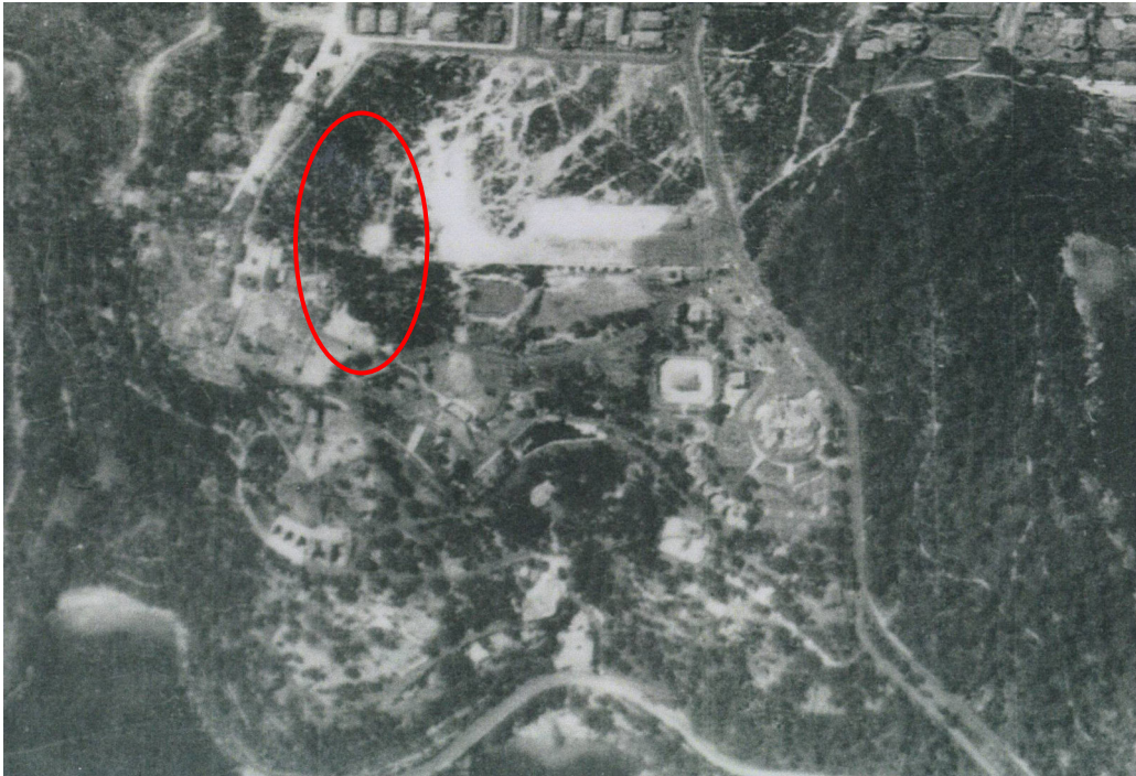
Photo 1 – Aerial photograph from 1930
