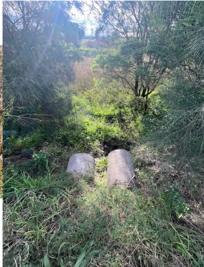
2 x 450mm dia Road Crossing
