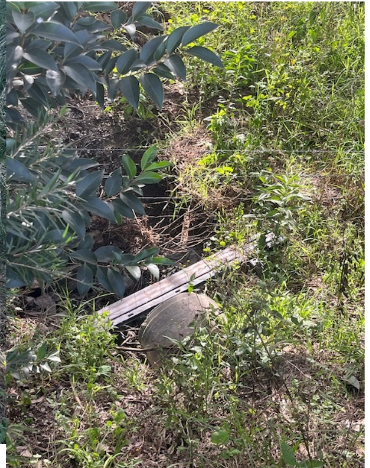
1 x 375mm dia Road Crossing
