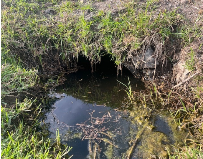
1 x 525mm dia Road Crossing
