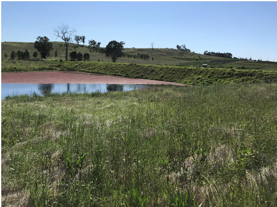
Photo 12 - Existing Fill around the dam, northeastern corner of the property
