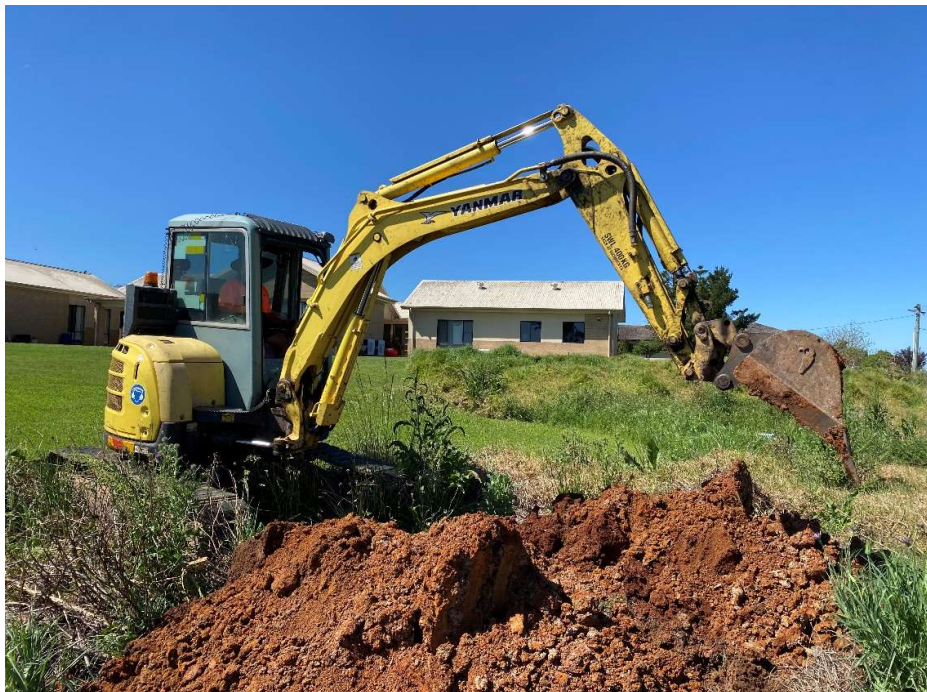
Photo 8 - 5 tonne excavator at TP08 (22/09/2020)
