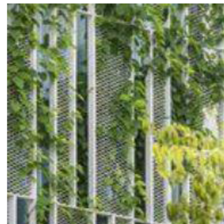
PERFORATED METAL WITH GREEN WALL
