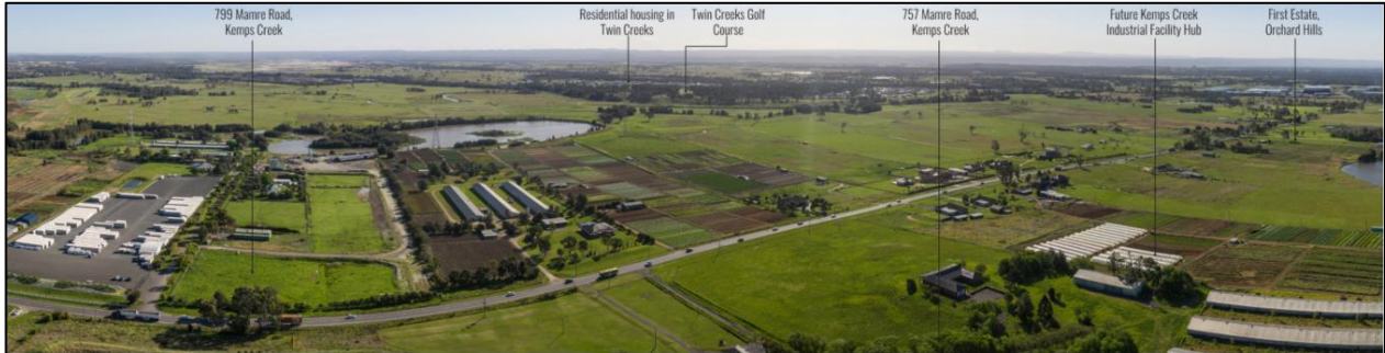
Figure 6 Existing site conditions - Looking west from Site's southwestern portion (Geoscapes 2021)
