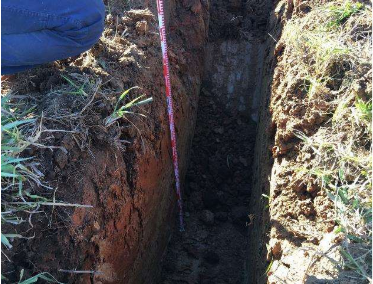
Test Pit TP23
