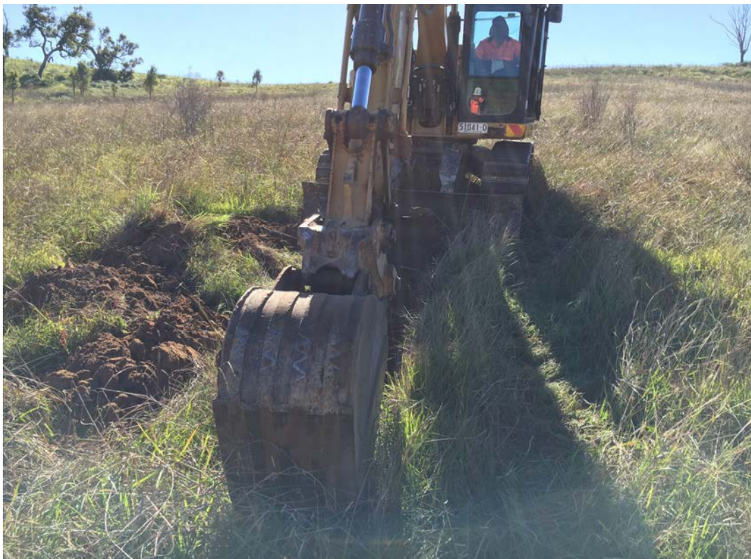
Photo 8 - 15T Excavator with the 500 mm Bucket
