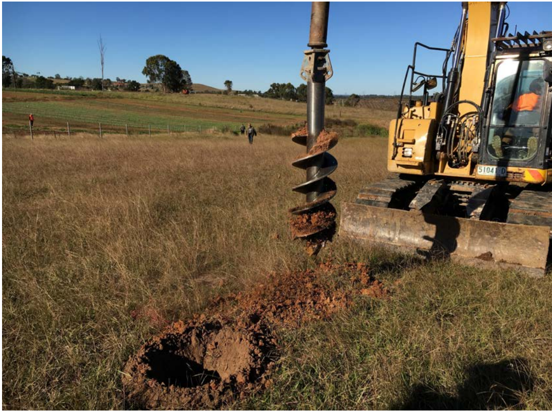
Photo 7 - 15 T Excavator with the 300 mm Auger
