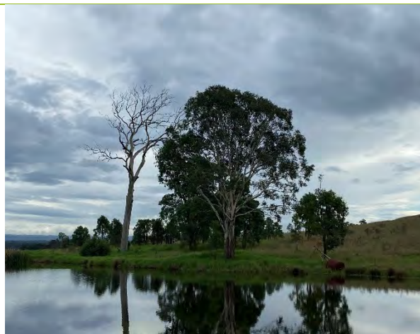
Photo 1. PCT 835 viewed from east side of dam
