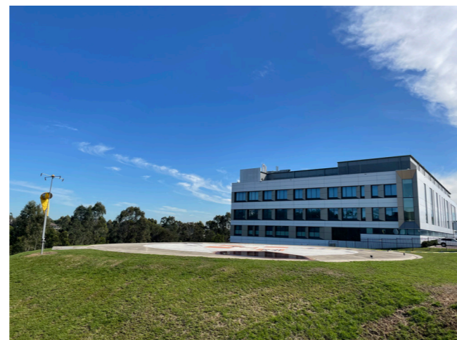
A View of Site from MCS towards Building D
