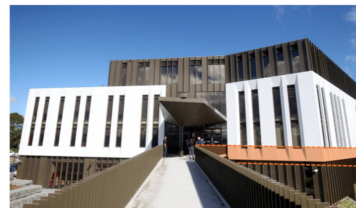
MCS BRIDGE LOCATION
