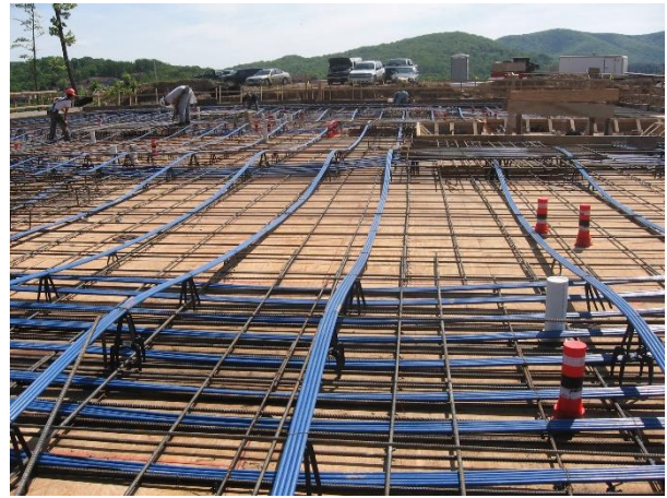
Figure 6 - Typical PT Slab under construction
