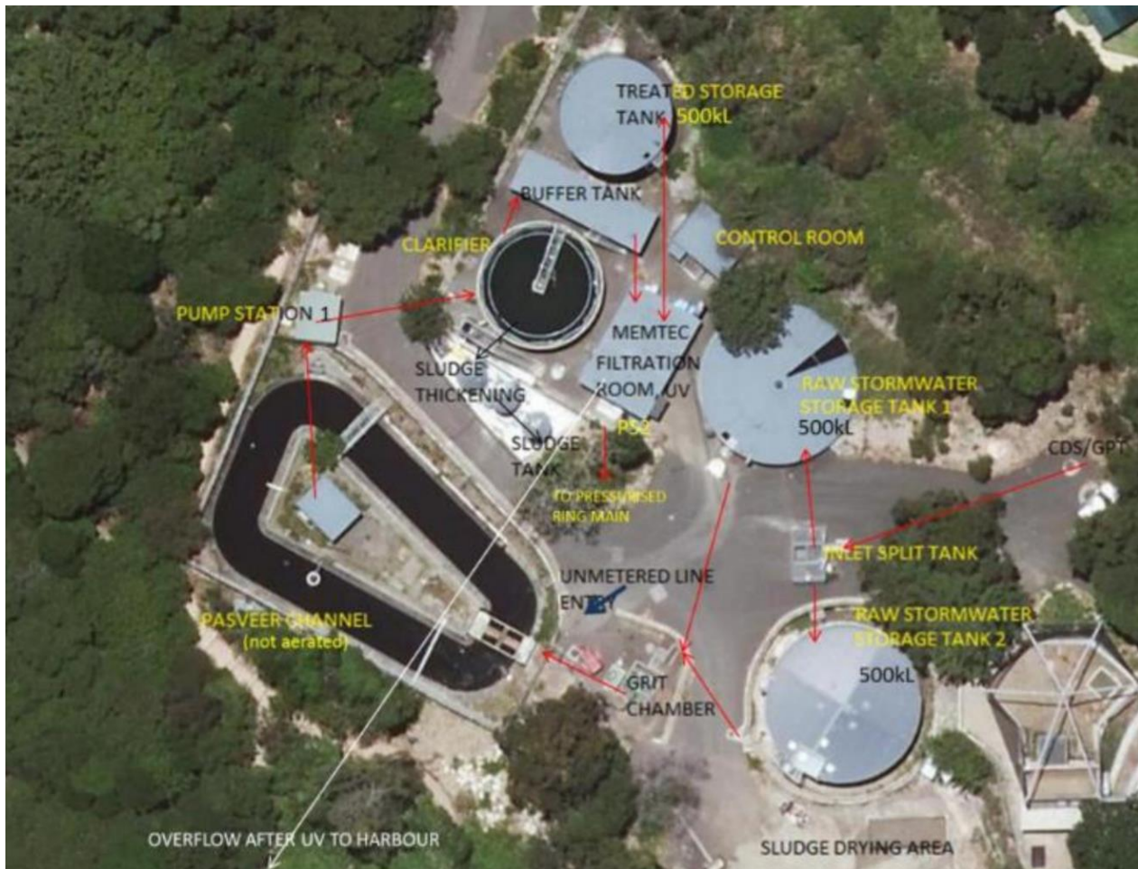
Figure 17 – Existing Waste Water Treatment Plant
