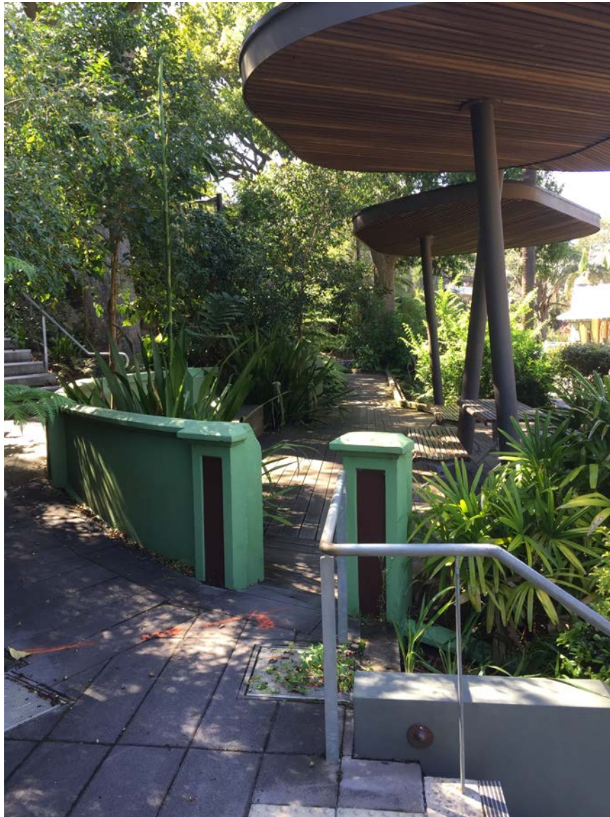
Figure 27 A 2021 view to the smaller 'D-shaped' aviary remnants with the most recent structures and floor decking within (designed and documented by Lahznimmo architects in 2009). The 1910s space has been repurposed as a rest/picnic area with the organic 'cloud-shaped' shelter canopies also acting as a quasi interpretation of the former aviary superstructure. The present picnic/shelter access arrangement retains the narrow former aviary keeper's access between the two piers. The stepped access in the foreground represents a recent upgrade (for BCA compliance purposes) to the convenient access provided between the two 'D-shaped' aviary remnants. As evident in this photograph, the steps allow access through to other steps leading to the upper road and floral clock lawn while the on-grade access through the smaller 'D-shaped' aviary also continues through (background in photograph) to the upper road beyond.
