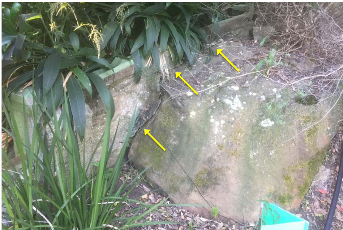
Figure 43 BELOW Detailed view of the western wall of the larger aviary showing its construction over and across (arrows) one of the natural rock outcrops in this area.
