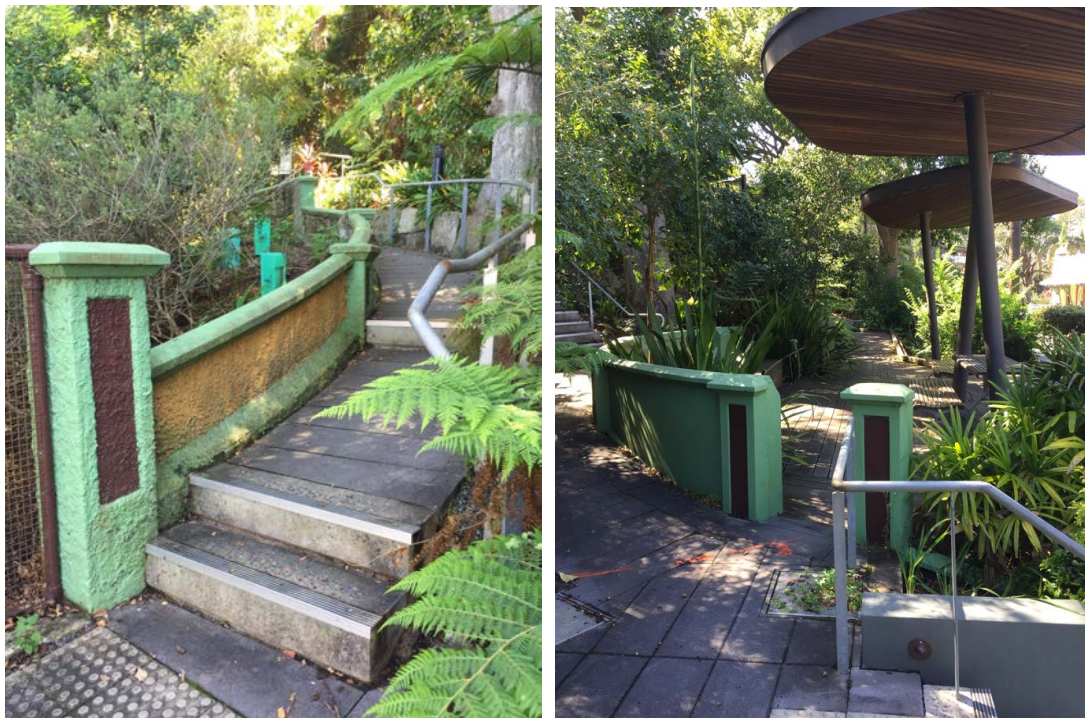
Figures 13 LEFT and 14 RIGHT show the present access arrangement that was introduced from the mid- 20 th century between, and partly around, the remnant 'D-shaped' aviaries.
