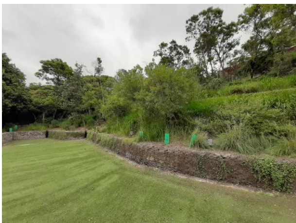
Figure 24 – The north-western portion of the subject area consists of steeply terraced gardens contained behind gabion walls.
