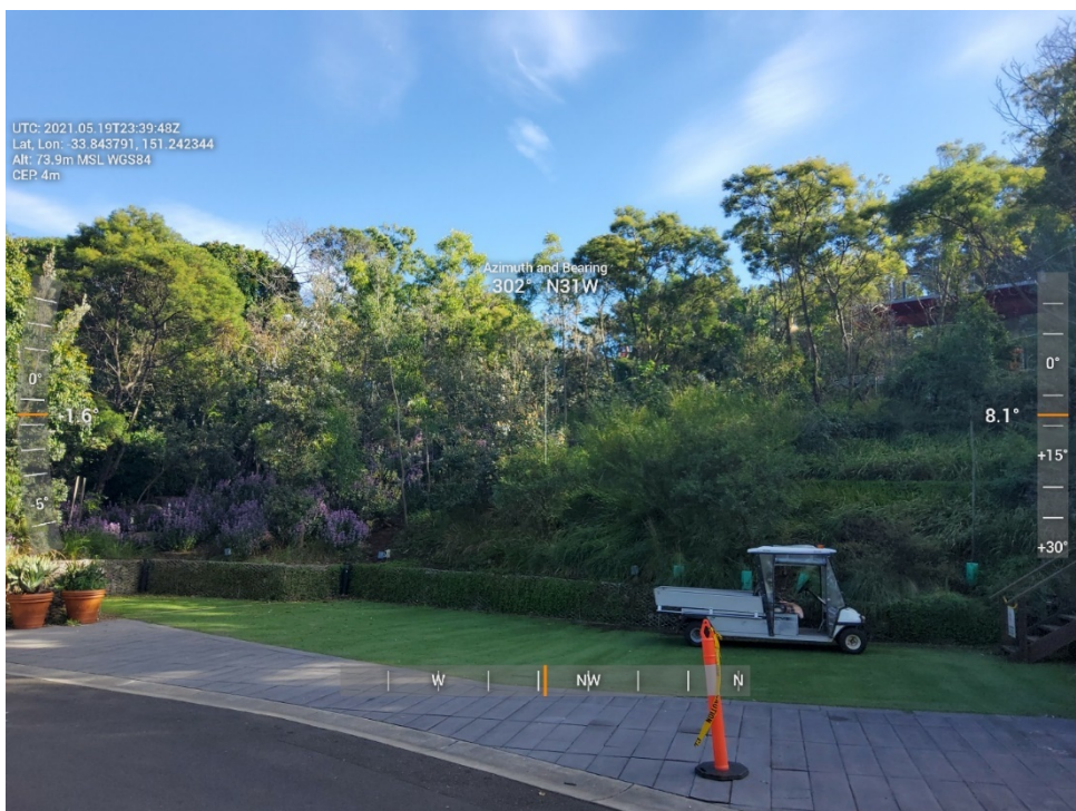
Photo 2.3: Looking north through the location of the proposed RACC. The project will involve the removal of most or all the vegetation behind the cleared area, with ramps and walkways proposed to be constructed from the terrace/walkway above/north of the RACC location (see Figure 2.1).
