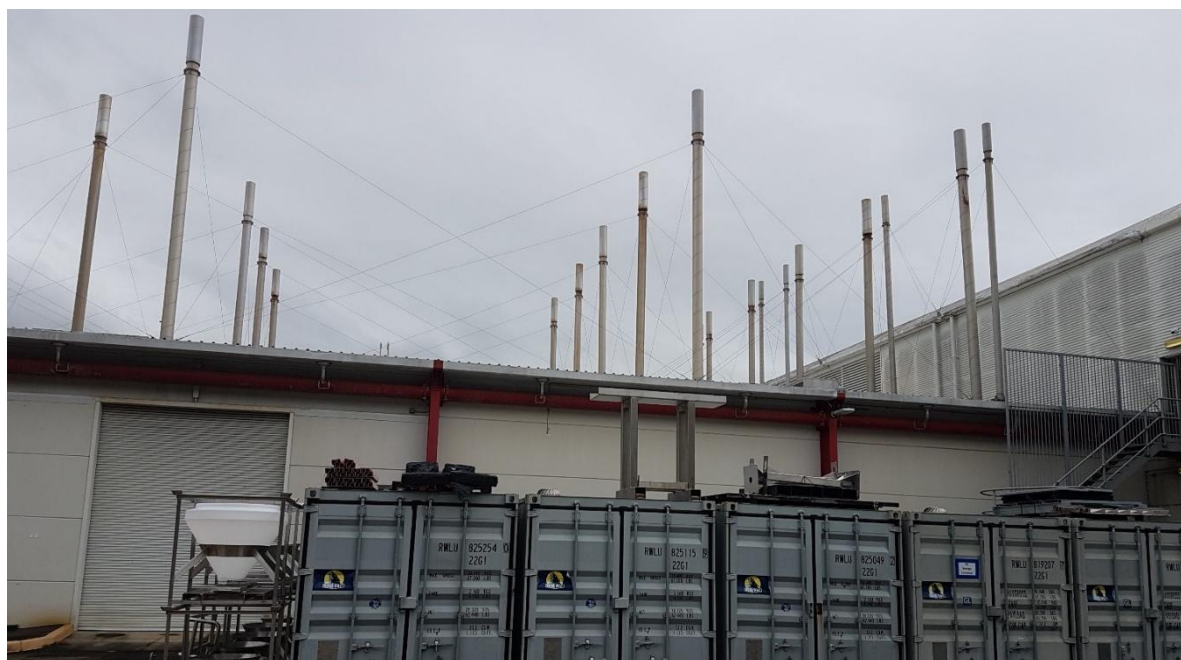
Figure 12 Photograph of Existing Bakery Building Showing Oven Stacks
