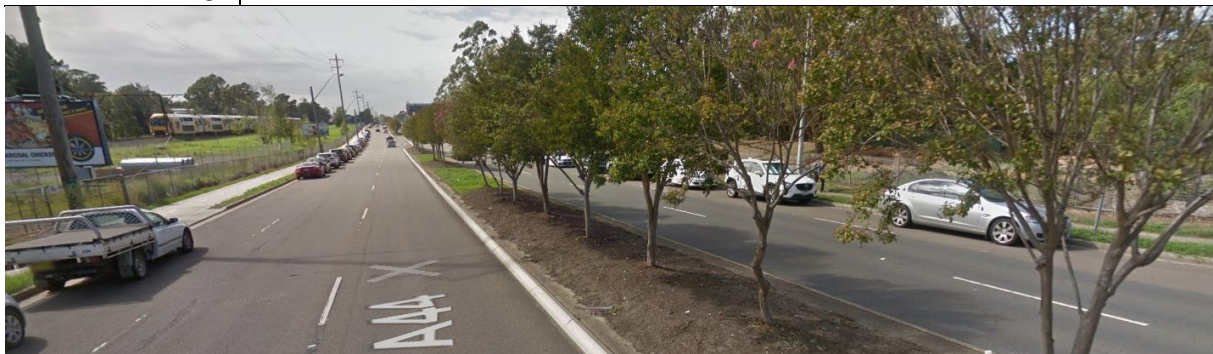
Figure 6 - Streetview of Great Western Highway, Eastbound (Source: Google)
